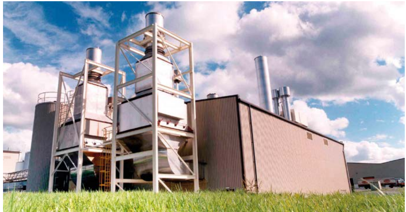
Power station at Mitchelstown, Ireland
