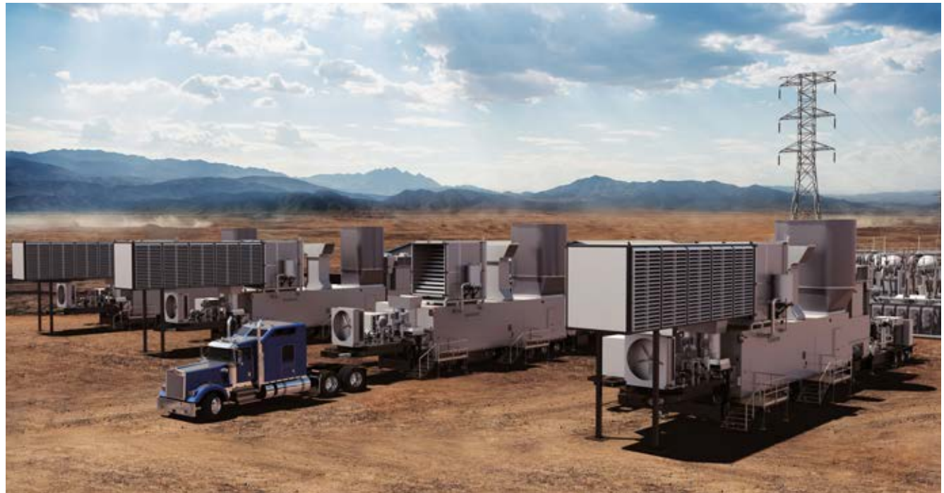
On-site installation of 4 SGT-A45 mobile units
