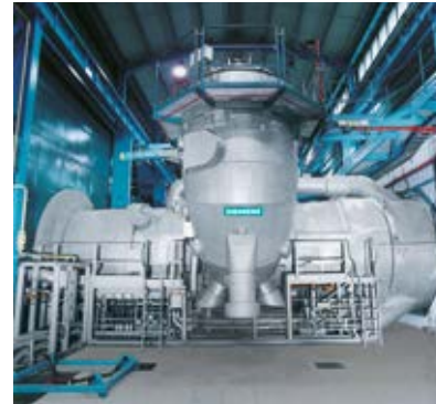
Excellent start-up and part load behavior, at up to 27 MW/min ramp rate
