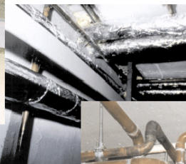
Insulation thicker than required by heating systems ordinance
