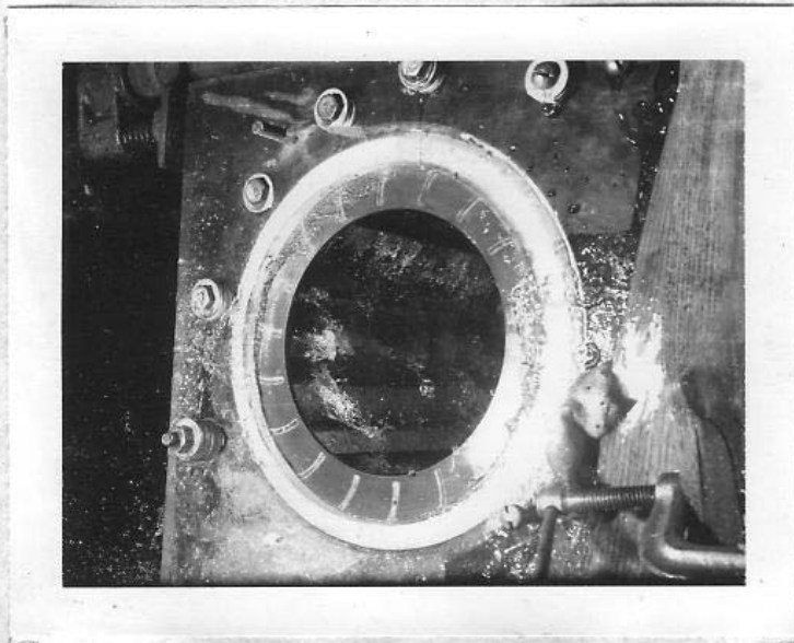
Photograph No. 6 - Original Nozzel
