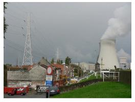
Figure 32.22 The people living near this nuclear power plant have no measurable exposure to radiation that is traceable to the plant. About 16% of the world's electrical power is generated by controlled nuclear fission in such plants. The cooling towers are the most prominent features but are not unique to nuclear power. The reactor is in the small domed building to the left of the towers. (credit: Kalmthouts)
