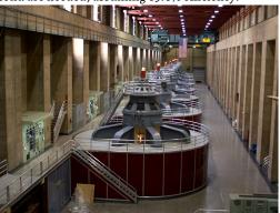
**Figure 20.43** Hydroelectric generators at the Hoover dam. (credit: Jon Sullivan)
