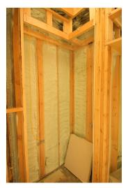
Figure 14.13 Insulation is used to limit the conduction of heat from the inside to the outside (in winters) and from the outside to the inside (in summers). (credit: Giles Douglas)
