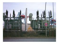
Figure 20.19 Power is distributed over large distances at high voltage to reduce power loss in the transmission lines. The voltages generated at the power plant are stepped up by passive devices called transformers (see <u>Transformers</u>) to 330,000 volts (or more in some places worldwide). At the point of use, the transformers reduce the voltage transmitted for safe residential and commercial use. (Credit: GeorgHH, Wikimedia Commons)
