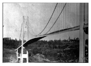
Figure 16.28 In 1940, the Tacoma Narrows Bridge in Washington state collapsed. Heavy cross winds drove the bridge into oscillations at its resonant frequency. Damping decreased when support cables broke loose and started to slip over the towers, allowing increasingly greater amplitudes until the structure failed (credit: PRI's *Studio 360*, via Flickr)
