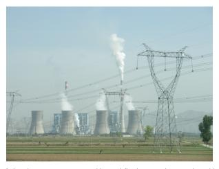
Figure 7.24 Tremendous amounts of electric power are generated by coal-fired power plants such as this one in China, but an even larger amount of power goes into heat transfer to the surroundings. The large cooling towers here are needed to transfer heat as rapidly as it is produced. The transfer of heat is not unique to coal plants but is an unavoidable consequence of generating electric power from any fuel—nuclear, coal, oil, natural gas, or the like. (credit: Kleinolive, Wikimedia Commons)
