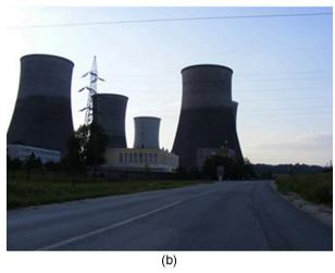
Figure 15.24 (a) A nuclear power station (credit: BlatantWorld.com) and (b) a coal-fired power station. Both have cooling towers in which water evaporates into the environment, representing  $Q_c$ . The nuclear reactor, which supplies  $Q_h$ , is housed inside the dome-shaped containment buildings. (credit: Robert & Mihaela Vicol, publicphoto.org)
