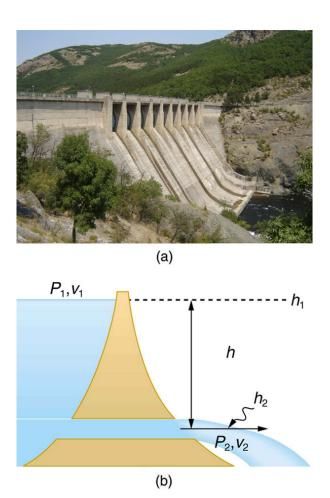
Figure 12.8 (a) Water gushes from the base of the Studen Kladenetz dam in Bulgaria. (credit: Kiril Kapustin; http://www.ImagesFromBulgaria.com) (b) In the absence of significant resistance, water flows from the reservoir with the same speed it would have if it fell the distance h without friction. This is an example of Torricelli's theorem.
