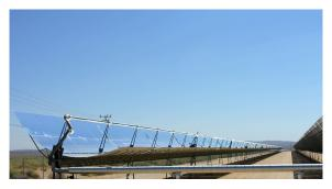
Figure 25.44 Parabolic trough collectors are used to generate electricity in southern California. (credit: kjkolb, Wikimedia Commons)
